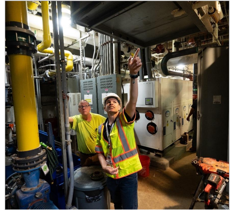
Reston Community Center Heating System Upgrade
